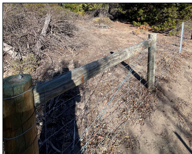
Figure 23: Onsite fencing infrastructure to limit disturbance for vegetation at RB Connolly Reserve.
