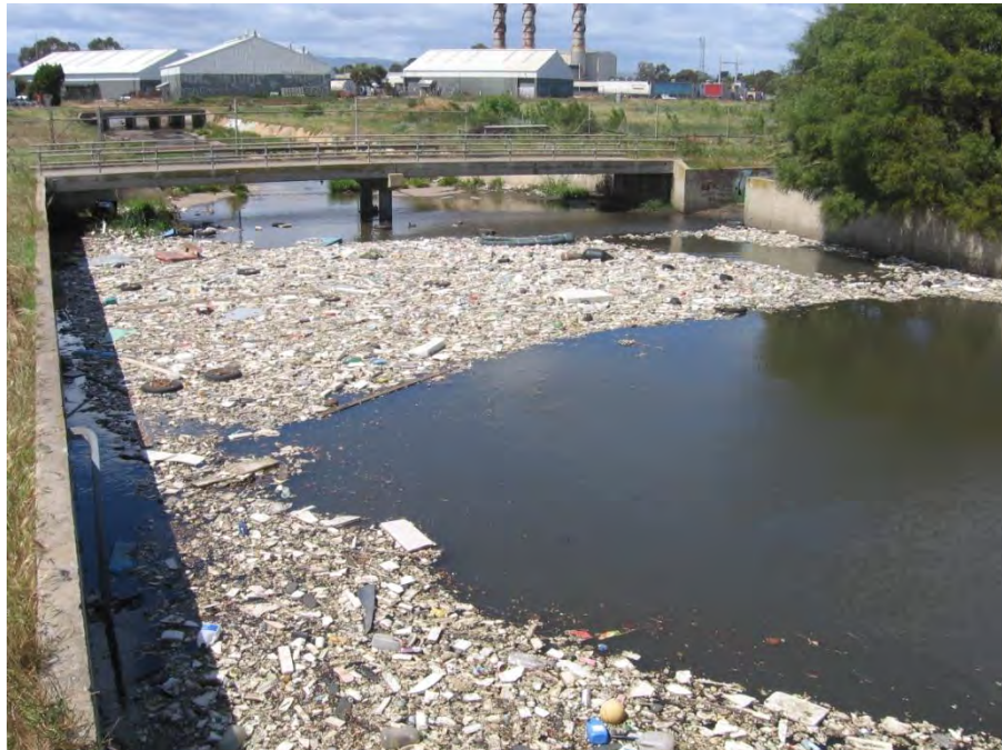
Figure 4.2: Build-up of debris behind the sewer siphon along the main outfall channel
