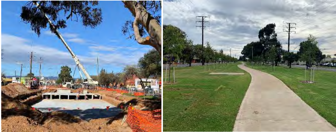
Figure 4.15 – Example of underground detention storage – during construction (left) and post-construction (right), (Port Road, Southfront 2019)
