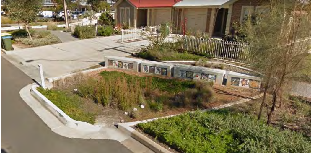
Figure 5.7—Bioretention System (Raingarden), Murchison Street, Woodville Gardens
